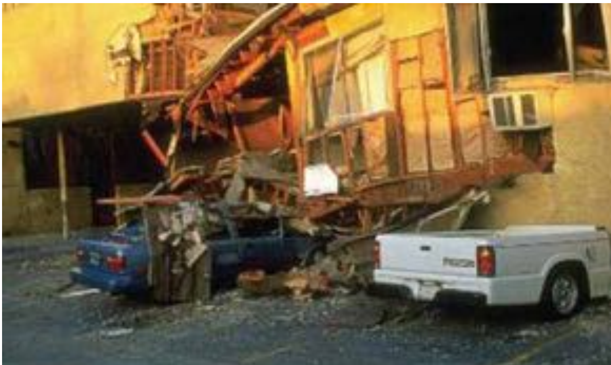
Figure 21: Tuck under parking and effects caused by Northridge earthquake (see USGS General Information Product 15).
